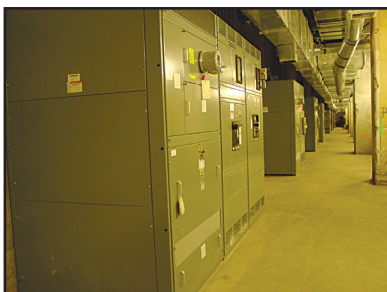
50,000 amps of 480 volt switchboards. Largest private electrical vault in Southern California
